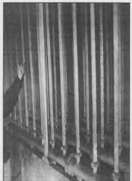
Photo: Air cleaner pipes, (nozzles are removed) and waste trough.
